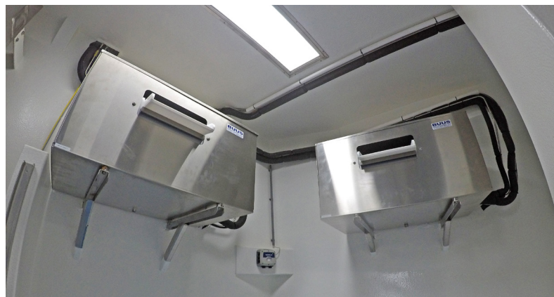
▲ Two Buus ice makers feed the ice pound with flake ice.
